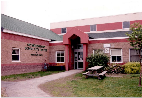
Seymour Osmon Community Center and Youth Safe Haven, ( New addition on the left )
